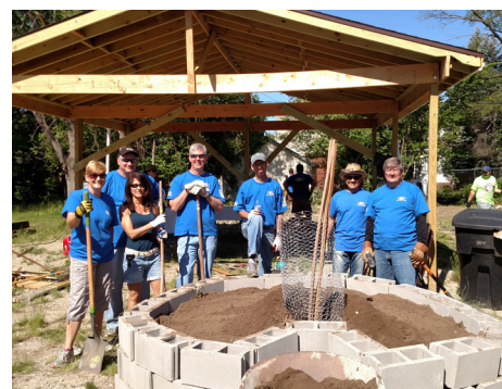
Employees from the Ford Motor Company helping to construct a rain garden with Popp's Packing. PHOTO BY MICHIGAN COMMUNITY RESOURCES.
