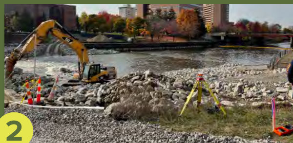
2 With the University of Michigan-Flint campus in the background, work crews remove crumbling concrete and place rock at the site where the dam once stood. Photo courtesy of EGLE.
